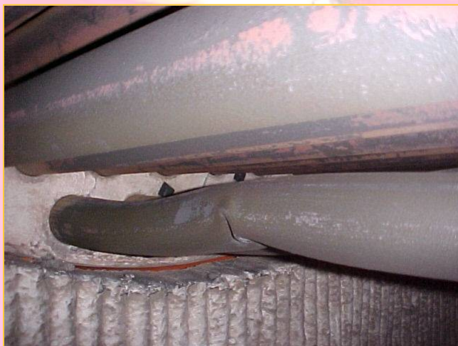
View of Pipe Directly Adjacent to Inlet Hot Combustion Gases
