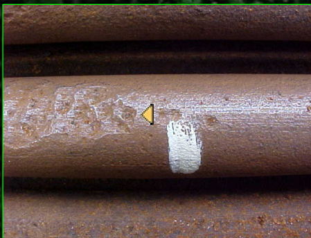
Isolated and interconnected pit sites
