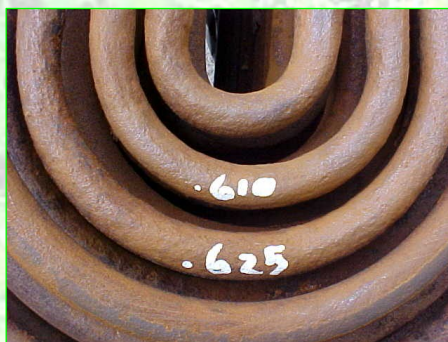
View of top periphery u-bends adjacent to inlet piping
