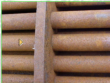
Tube and support condition away from corrosion zone
