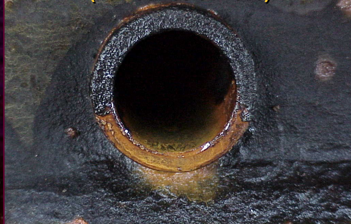
Original thickness tube in outlet pass (non-corrosion zone)
